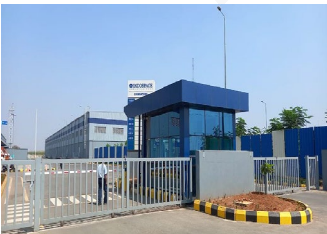
Fabric warehouse at Tirupur
