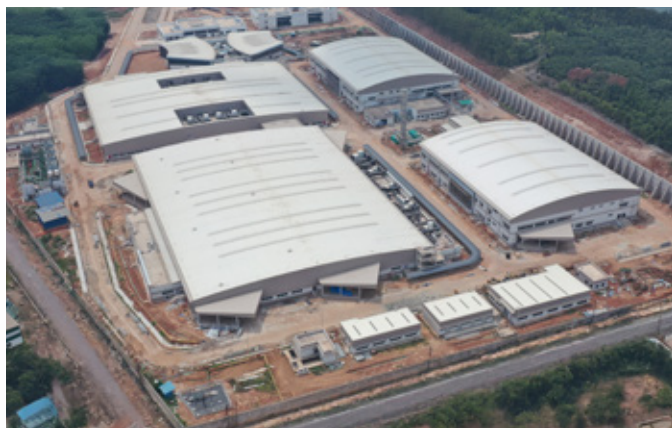
New Manufacturing plant at Odisha
